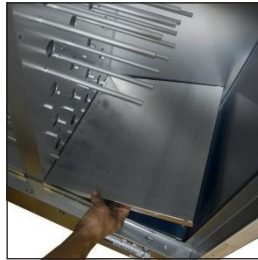
A3. Remove aluminum finishing panels
